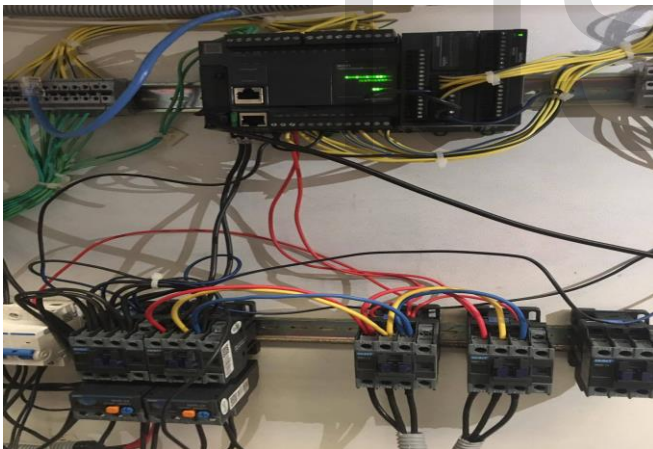
Fig.4. Connection diagram showing PLC and contactors Schneider Electric Modicon TM221 Series is used. This series consists of two modules which are specified below: i. Module 1: TM3DM24R/G ii. Module 2: TM3AM6/G
